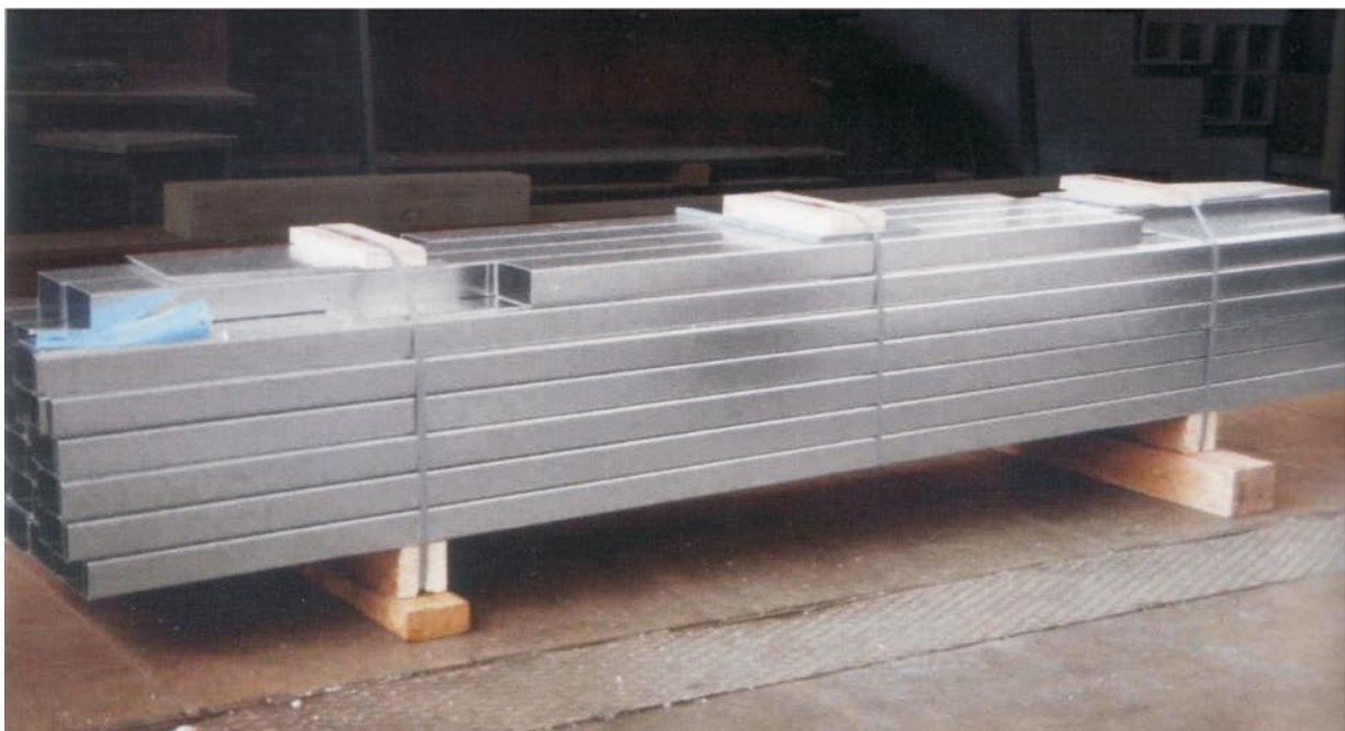
Storage of packages from the profiles ensuring slight slope
